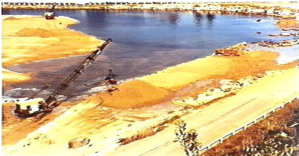
Figure 53 Council clearing the entrance of the lagoon 1982
