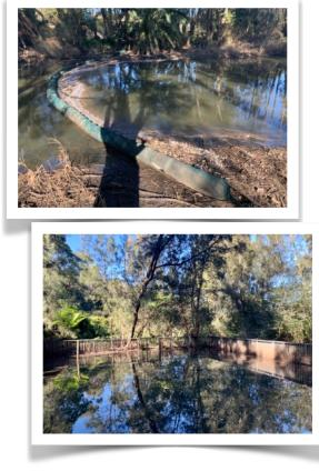
There are 26 Gross Pollutant Traps (GPTs) around the Manly Lagoon Catchment, with only 16 on a regular or semi regular cleaning schedule. Council removes around 900 tonnes of waste from them each year and is working towards improving maintenance schedules.
